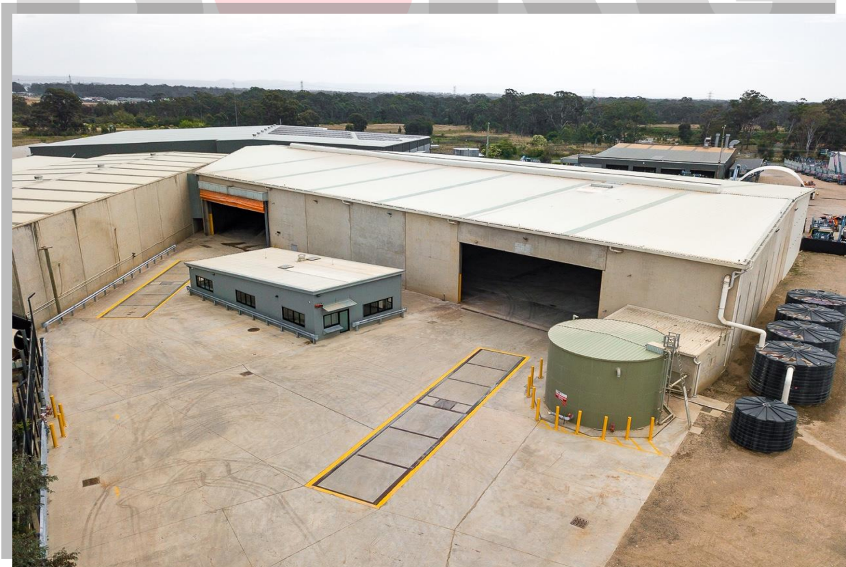
Photograph 1- Existing buildings on 25 Dunheved Circuit, St Marys
